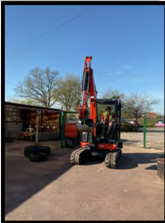
Talia's Dad's Digger.
